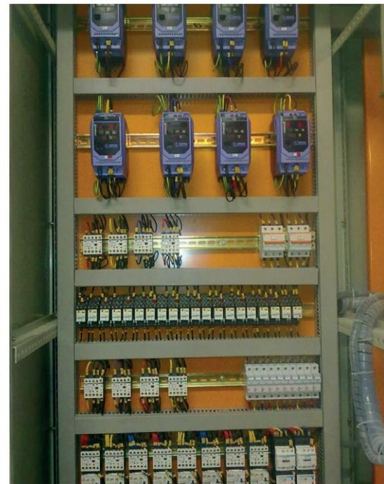
Optidrive E2 single phase output is designed for use with PSC (permanent split capacitor) or shaded-pole single phase induction motors with IP 20, IP 55 and IP 66 enclosures.
