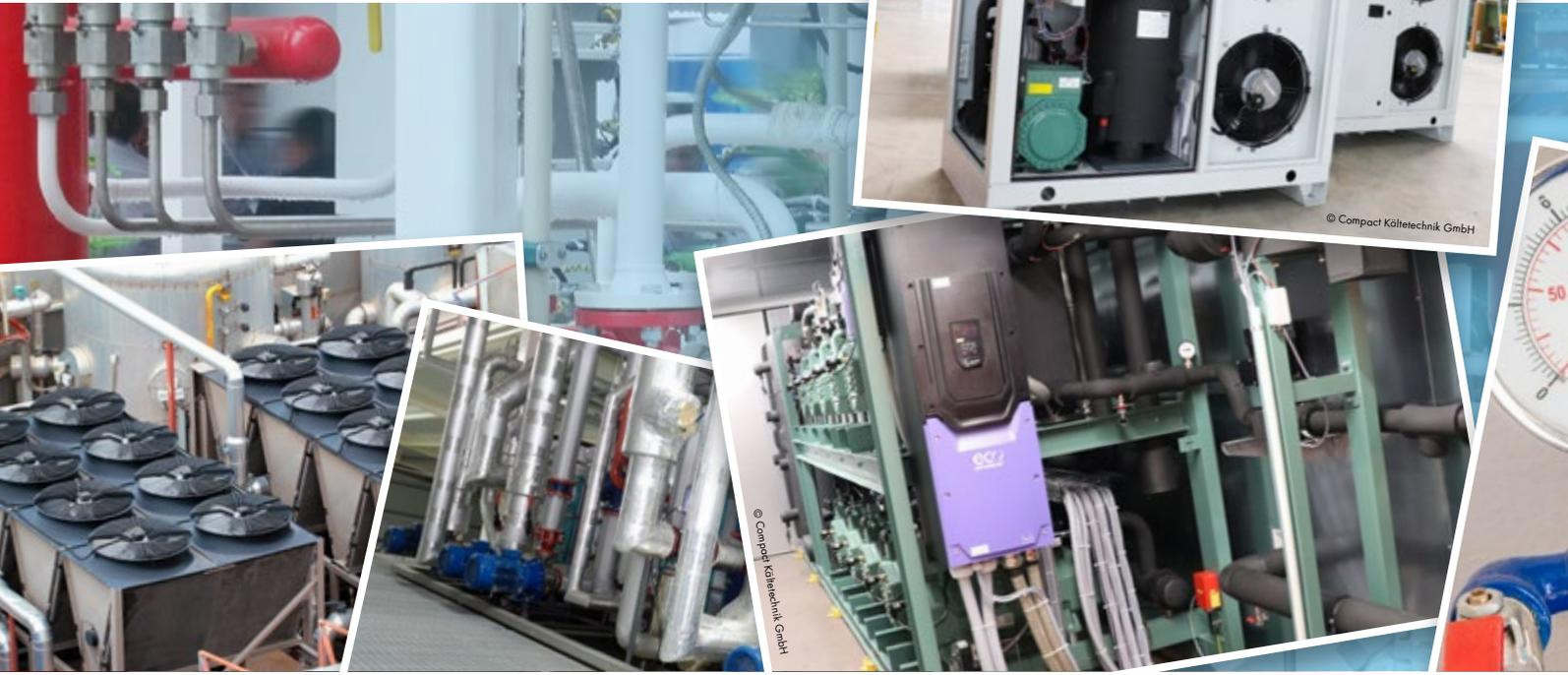
Installation of **OPTIDRIVE™** variable frequency drives to control refrigeration compressors, significantly reducing energy consumption, and improving system COP (coefficient of performance)
