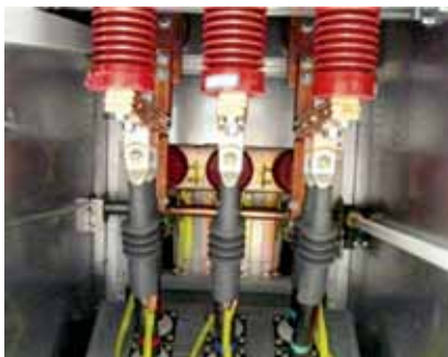
Connected power cable to the feeder busbar
