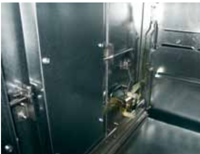
Interlock for circuit breaker compartment door
